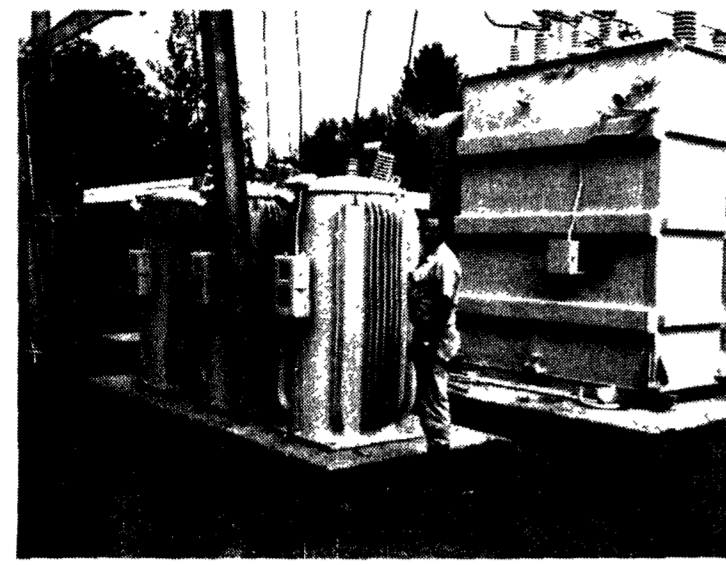
Commissioner Al Fletcher beside automatic voltage regulator. 10,000 KVA transformer in background.
